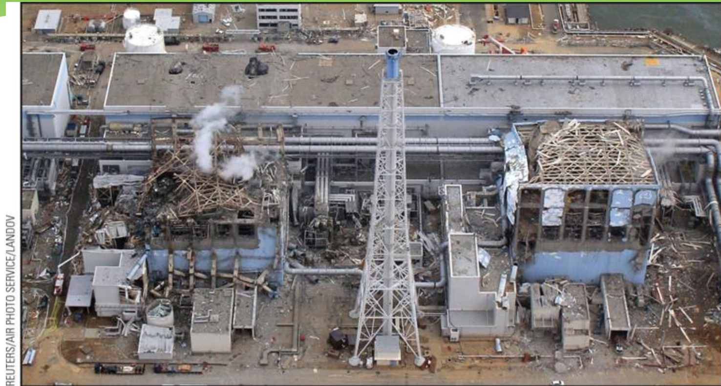
Figure 6.26: Damage to Fukushima Dai-ichi nuclear facility reactors 3 (left) and 4 (right) on March 20, 2011.
