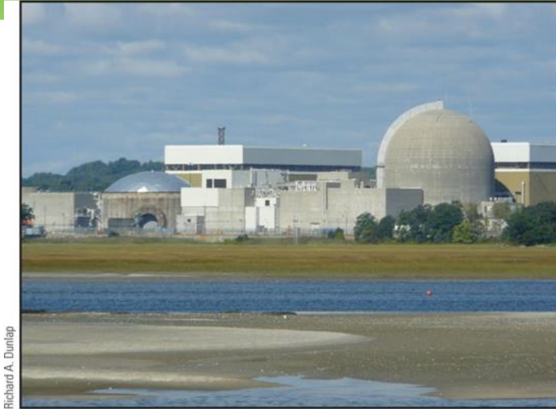
Figure 6.11: Seabrook Nuclear Generating Station in New Hampshire U.S., a 1244-MW e PWR. The reactor core is contained inside the dome-shaped containment building at the right.
